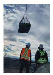
During the process, the helicopter performed approximately 30 lifts over five hours. The five-hour time span allowed the steel base of the structure to be carried, assembled, and welded on the roof before the landing of the cooling towers.
