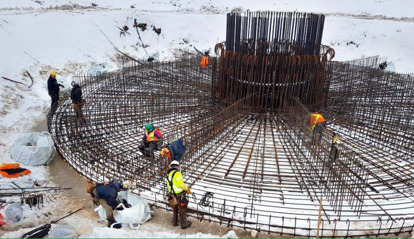
B&M team members erect a turbine base on site in Riverside-Albert, NB.
